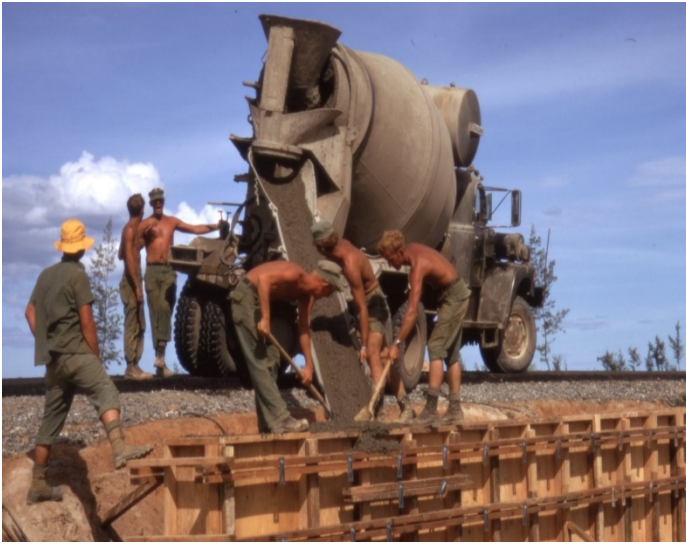
Upper left MCB- 62 bridge abutment pour, Upper right MCB-7 Rock Crusher. Contributors unknown and dates.
